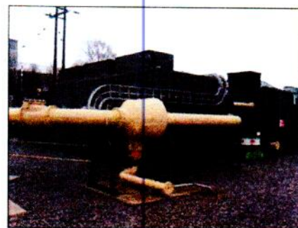
15" KSS Cyclone Separator Natural Gas Application
